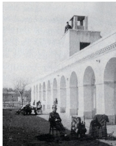
Machine gun post on roof.
